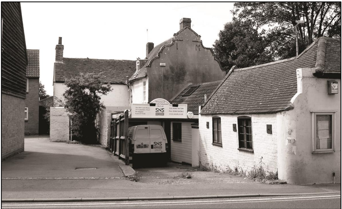
The blacksmith's forge, attached to the north gable of Grove House - 2006
